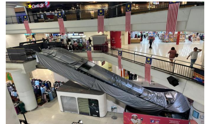
Installation of modernized escalators
